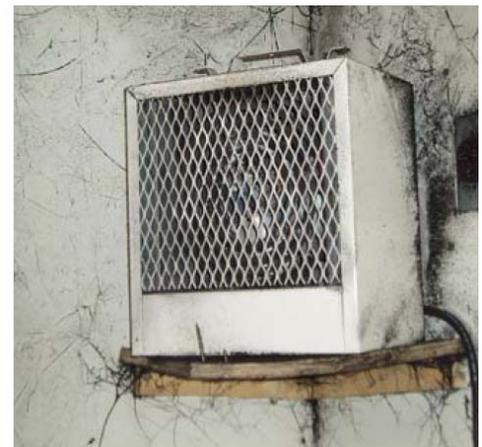
*Incorrect placement: heater's air exhaust is obstructed.*
