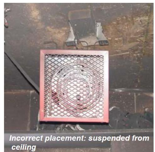
*Incorrect placement: suspended from ceiling*
